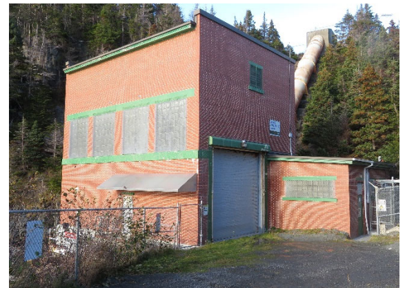
Cape Broyle Hydroelectric Generating Plant.
