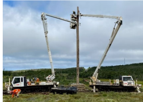
Single pole construction on transmission line 94L.
