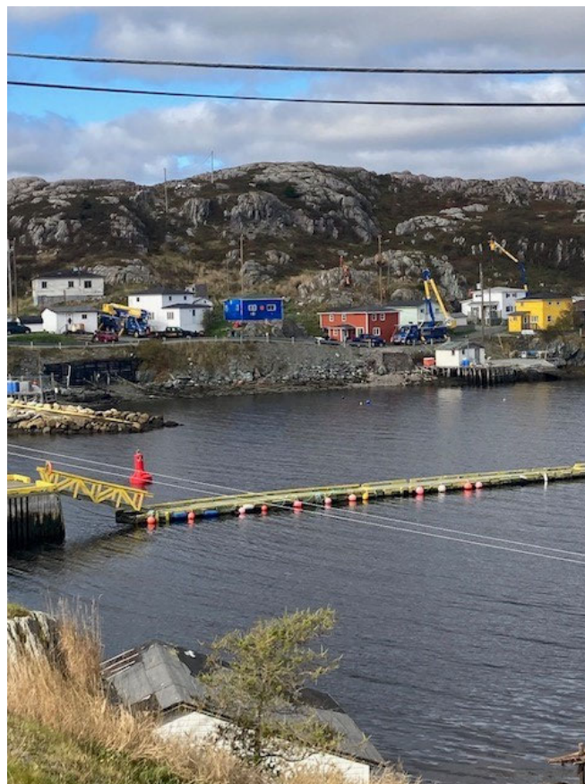
Crews replacing poles and conductor on BLA-01 in Harbour Mille.
