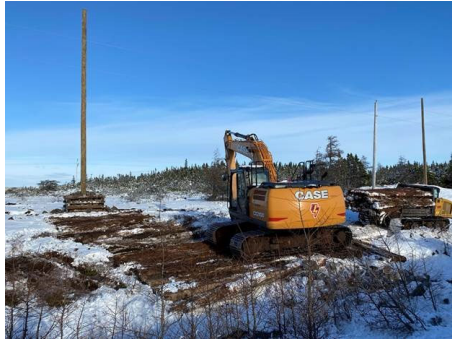
New pole installation on transmission line 55L.
